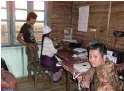
Fig. 39. The view inside the facility. In the foreground is the satellite phone and in the background a radio device for communicating with Mindat.
