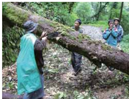
Fig. 3. Removing a fallen tree blocking the road to Hilong village. August 15, 2007.
