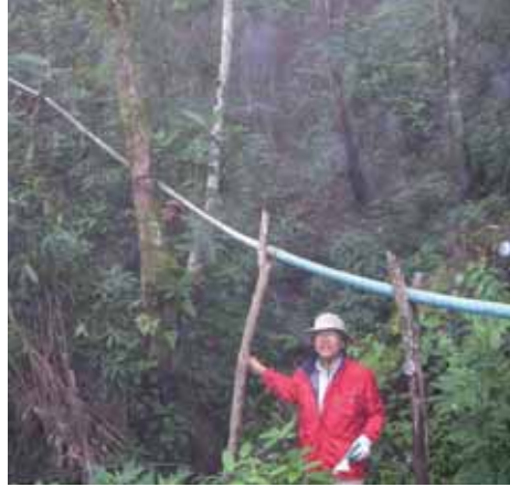
Fig. 56. PVC pipes are tied to trees or supported by forked branches to cross cliffs.
